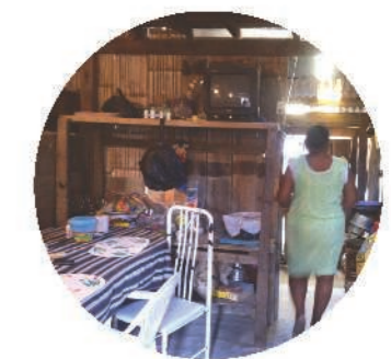
A TYPICAL DWELLING Bamboo structure and panelling
